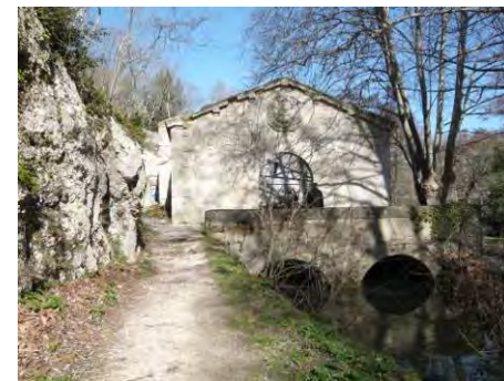
La station de pompage.
